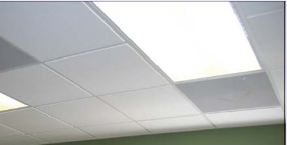
The interior of this building was painted by the factory with carpeting installed onsite. The ceiling is recessed reveal edge T-Grid with additional can lighting on dimmer switches in the conference room.
