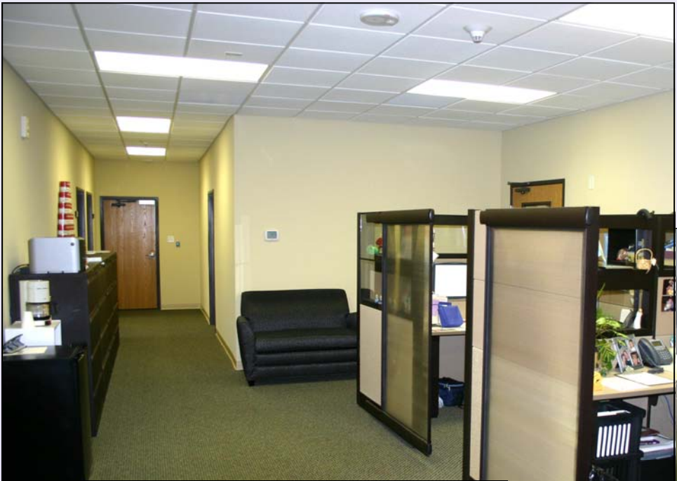
The interior of this building was painted by the factory with carpeting installed onsite. The ceiling is recessed reveal edge T-Grid with additional can lighting on dimmer switches in the conference room.
